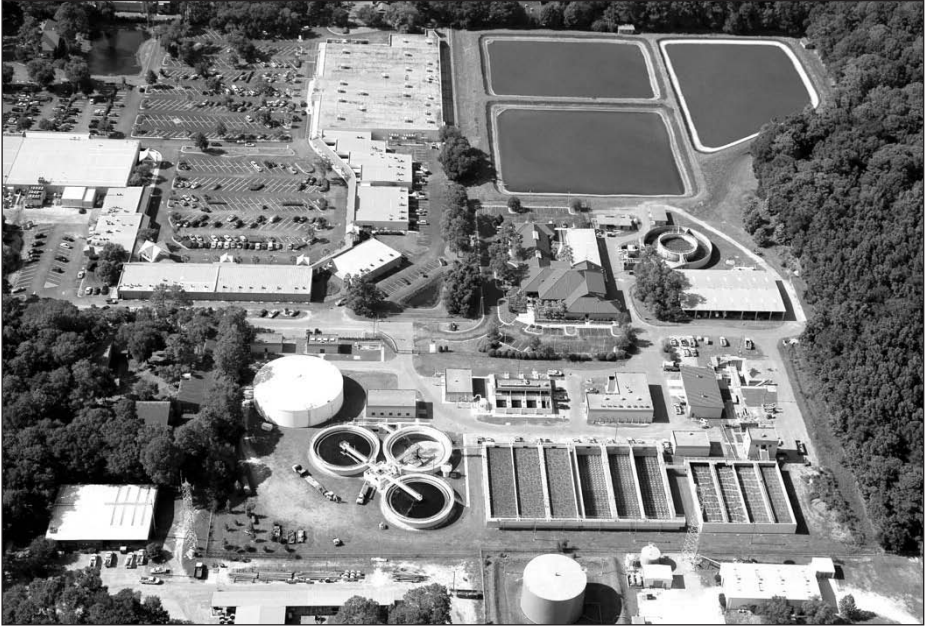
Hilton Head PSD is located at 21 Oak Park Drive, off Mathews Drive. This aerial photograph shows the PSD with Port Royal Plaza in the upper left corner.
