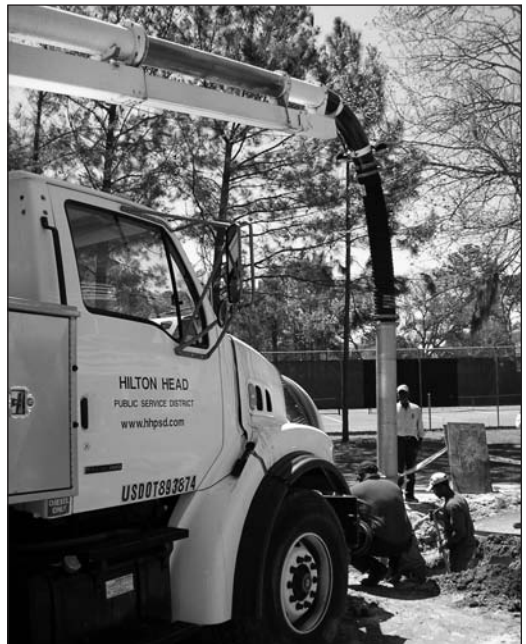
The PSD's Operations department uses its vacuum truck during repair projects.
