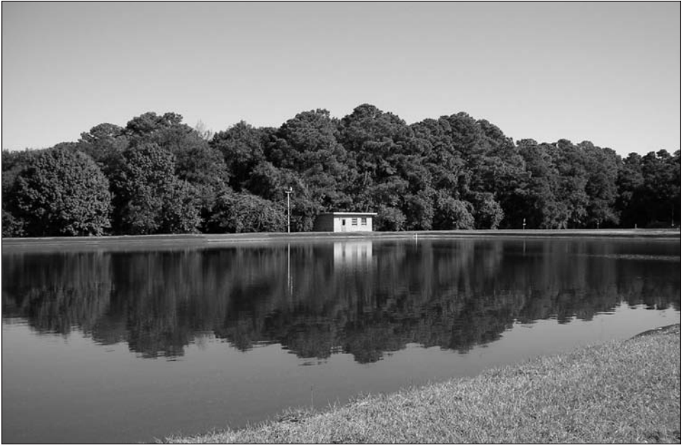
The PSD's Reclaimed Water lagoon can store 30 million gallons of highly-treated Reclaimed Water.
