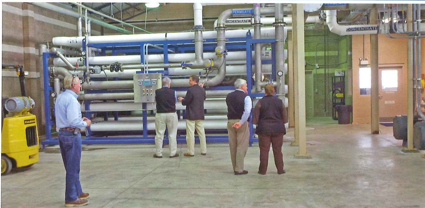
Edisto Beach officials toured the PSD's Reverse Osmosis (RO) Plant recently to learn about the process as they consider constructing a smaller plant for their community. Edisto Beach, like Hilton Head Island, is faced with lost drinking water supply as a result of saltwater intrusion into their groundwater source. The PSD's RO Plant is a key tool in the fight to replace supply lost to saltwater intrusion.
