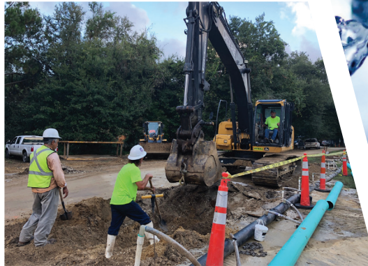
Recent sewer work along Bligen Lane
