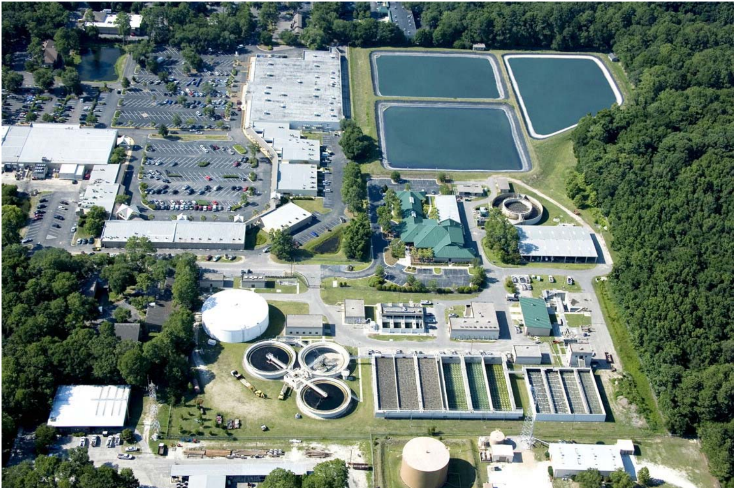
The Hilton Head PSD Water Resource Center & Recycled Water Plant, 21 Oak Park Drive, Hilton Head Island, SC
